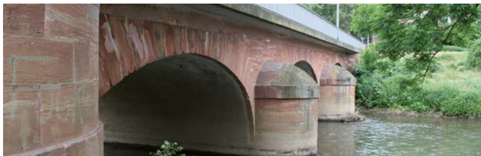
Niddabrücke in Nied
