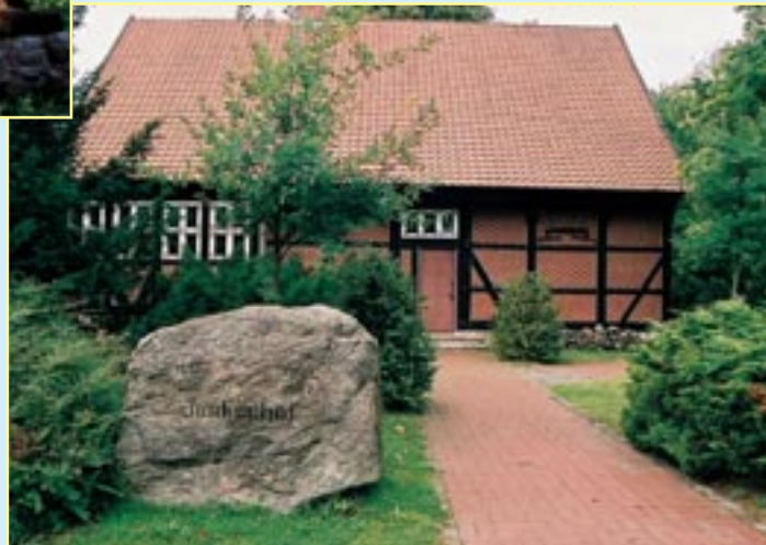
Junkerhof in Wittingen
