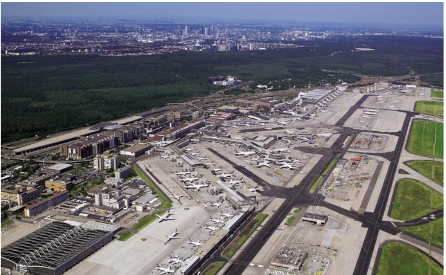
Rhein-Main-Airport, Frankfurt / Rhine-Main Airport, Frankfurt
