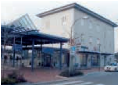
Bahnhof Railway Station
