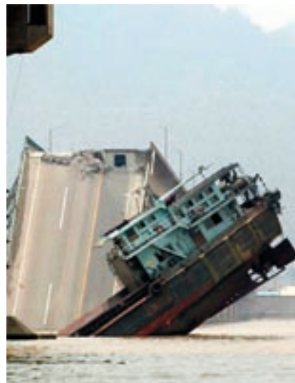
Figure 1: Collapse of the Jiujiang bridge after ship impact (2007 in China) and of the Murrah Federal Building in Oklahoma City (1995 in the USA)
