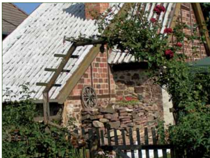
Backhaus am Friedrichshohenberg
