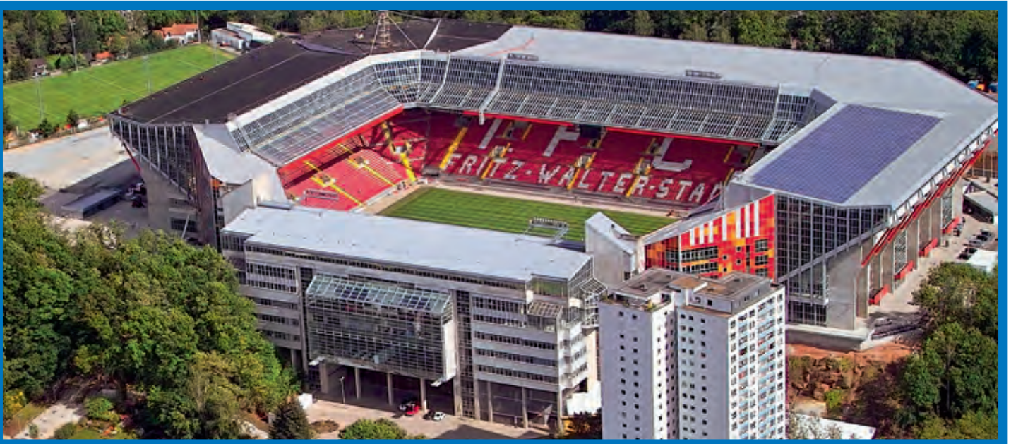
Fritz Walter Stadium
